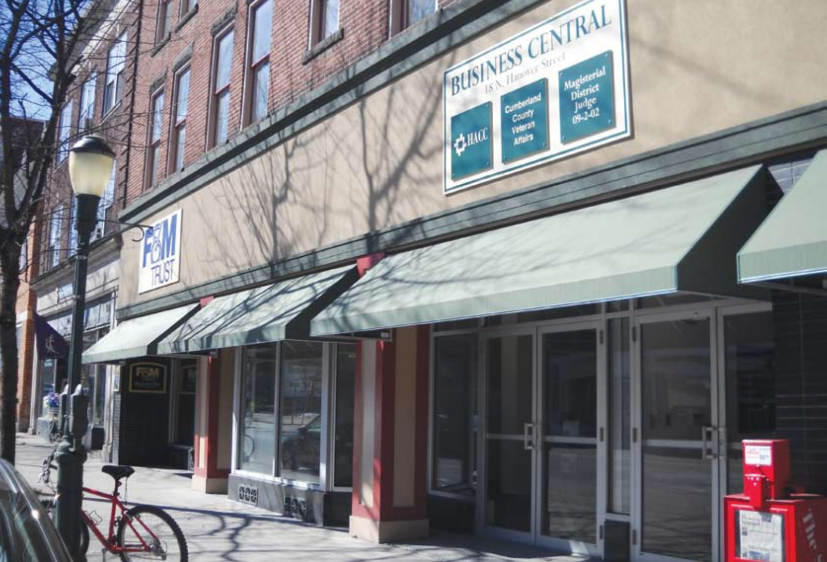
BUSINESS CENTRAL Using funds from four different sources, the Redevelopment Authority rehabilitated the former Woolworth's building for retail and commercial use
